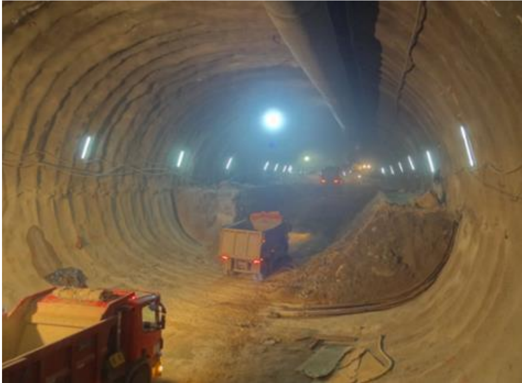
Diagram 3.6 Mining a Cavern Station
